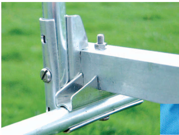
● Fig. 2: (above) Element clamps hold the elements to the boom. See text for more detail.
